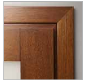
connection of architraves
